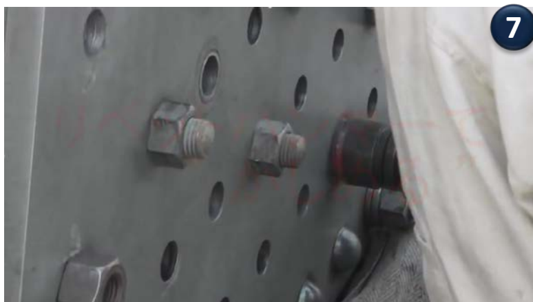
cool down during caulking
