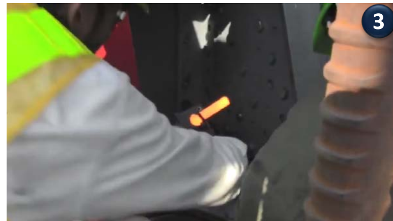
rivet into hole by hammer
