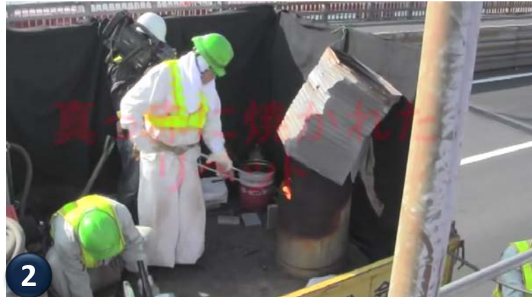
red riped rivet by 1200 deg.
