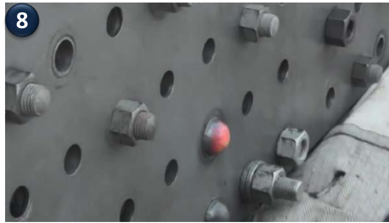
caulking almost finished
