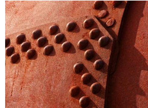
steel plate structure with rivet
